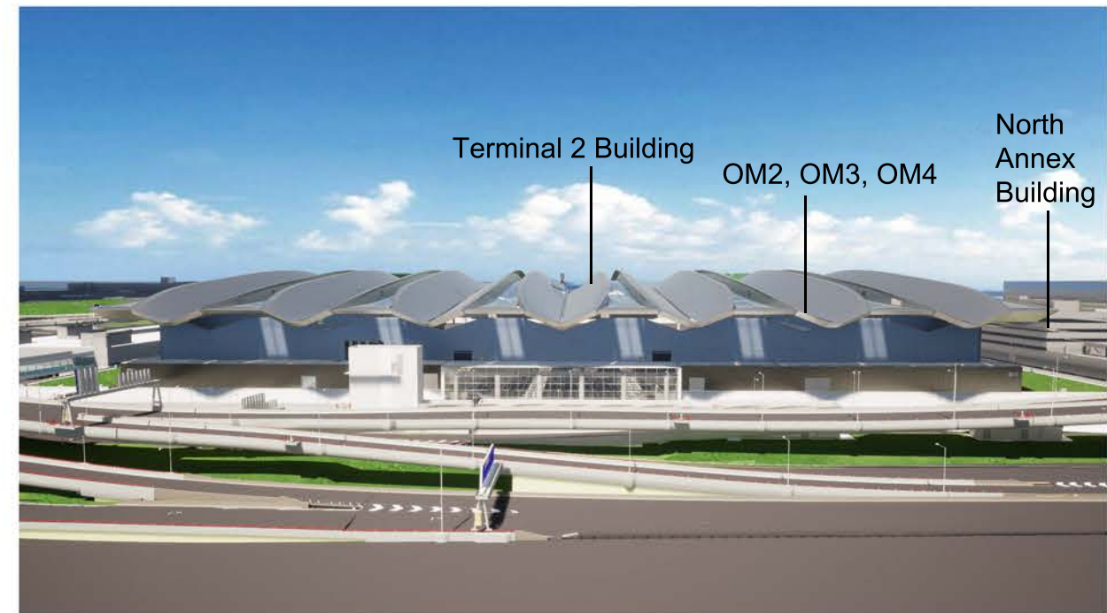
East side of Terminal 2 (T2) Building
